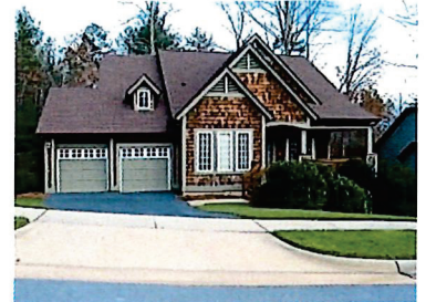
Single-Family Homes with Driveway
