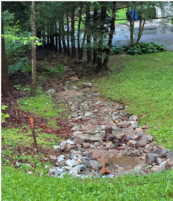
Photo of receiving ditch
