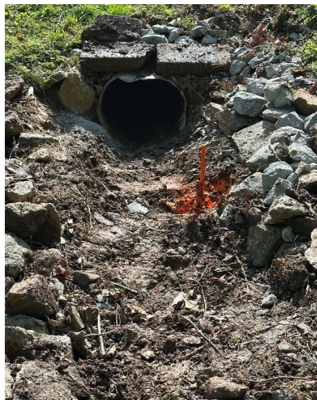
Photo of storm pipe with plug removed
